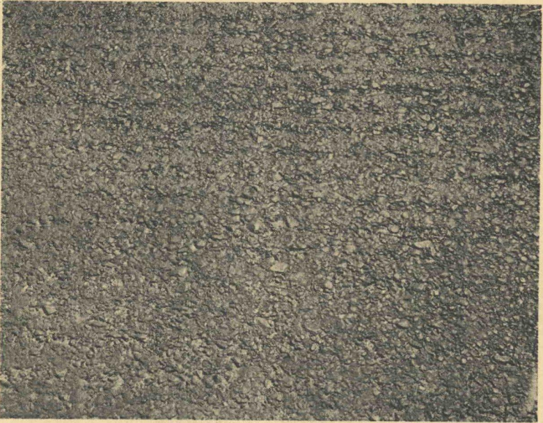
Figure 4. Pavement Surface Texture on Asphaltic Concrete Test Section (NS7 Run)
