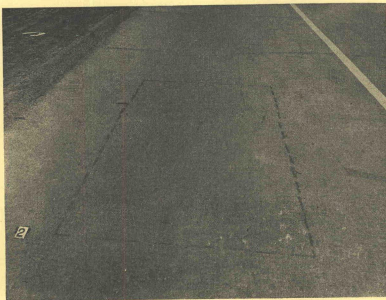
Figure 6. Route 2AB, Los Angeles County, California. Uniform four-inch resurfacing slab on four-inch base with 2\frac{1}{2} feet by 8-inch widening shoulder. Patch in old base, as indicated by dash lines, concreted monolithic with the resurfacing, has not caused cracking in the resurfacing.
