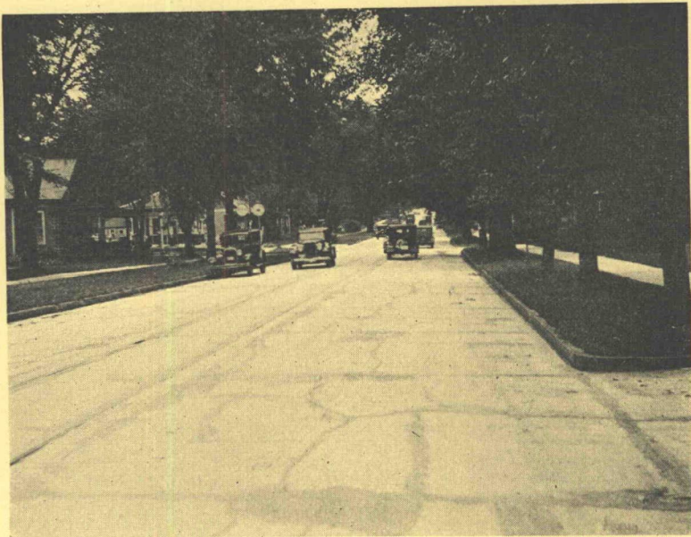
Figure 1. East Main Street, Marshalltown, Iowa. Resurfaced in 1911. Photographed 1932. Four-inch plain concrete on a five-inch natural cement concrete base. The railway track was built later and the pavement had to be cut out in the track area, which is blamed for much of the cracking in this twenty-one-year-old pavement.
