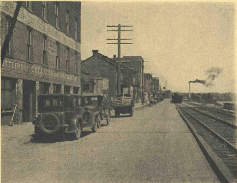
Figure 3. Water Street, Cape Girardeau, Mo. Resurfaced 1916. Photographed 1932—16 years old. Four inches of plain 1:1½:3 concrete on seven-year-old concrete base. In good condition except one broken area. Dray and truck traffic.
