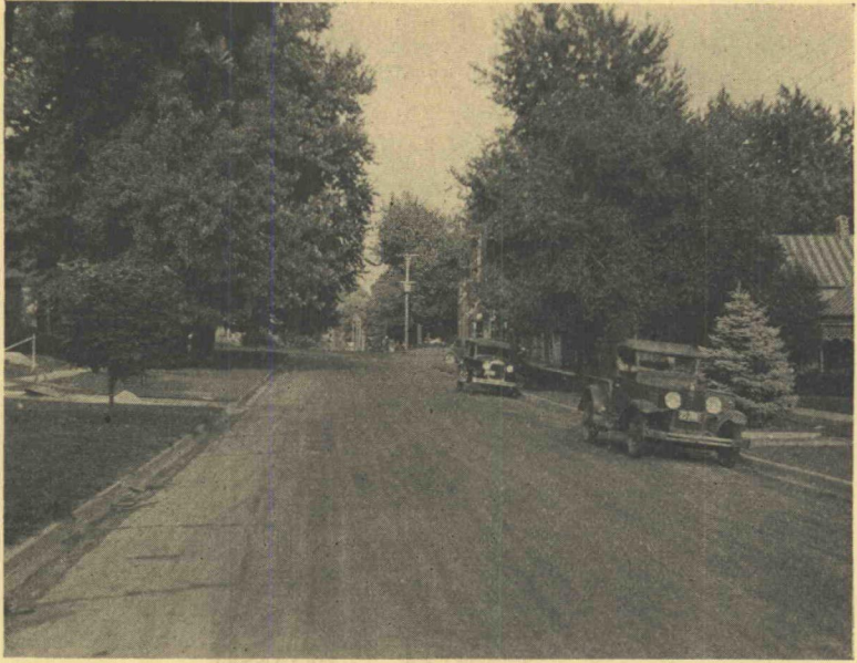
Figure 2. Market Street, Savannah, Mo. Resurfaced 1914. Photographed 1932—18 years old. Two-to-three-inch concrete over one year old concrete base. Light mesh reinforcement. Oil tracked onto pavement from oiled dirt streets. Cracked, but good for many years. Light traffic.
