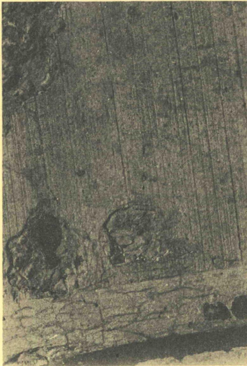
Figure 1. Lines of Disintegration in Concrete Slabs. Called " D " Lines
