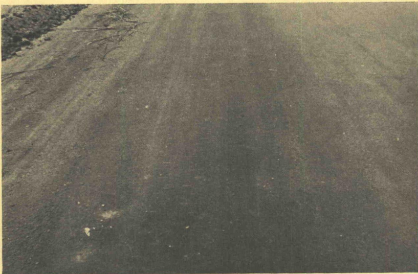
Figure 25. Close-up View of the Sand-Gravel Road Surface Treated with Calcium Chloride. Note the Absence of Loose "Float" Material. (Nebraska Project.)
