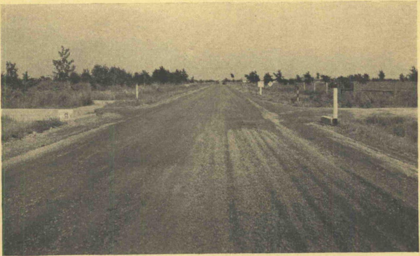
Figure 13. Junction of Test Road with Part Maintained in Regular Manner.
