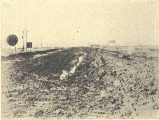
Figure 2. Typical Untreated Minnesota Gumbo Road Surface in the Early Spring.
