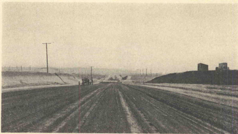
Figure 14. La Tijera Boulevard. Stabilized soil after completion of mixing. Mixed material was bladed out from roadway to form 3-foot V gutters
