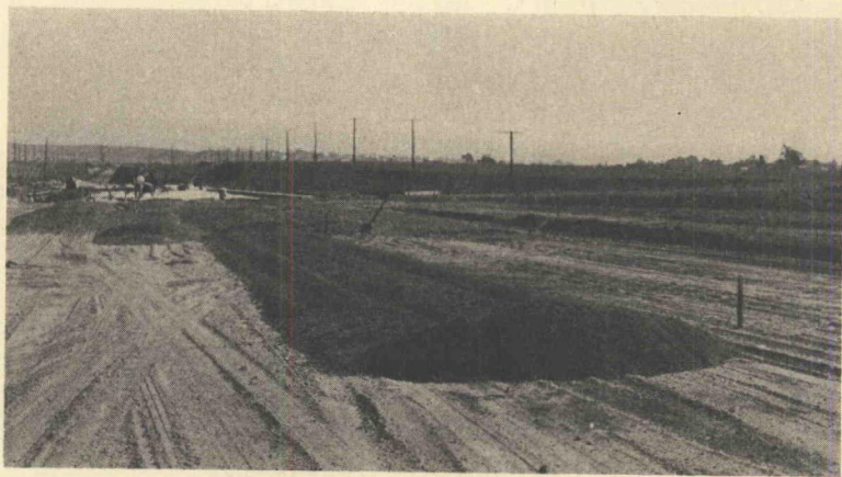
Figure 12. La Tijera Boulevard. Sand being spread for blending with clayey soil prior to stabilization
