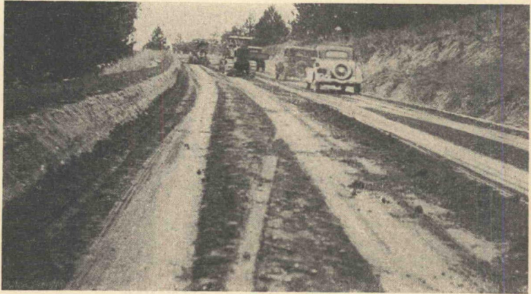
Figure 19. Project shown in Figure No. 18. Stabilized base was compacted under traffic
