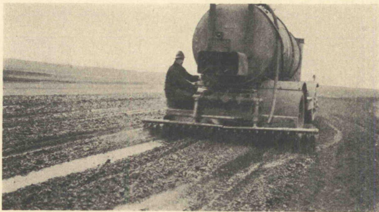
Figure 9. Glenn Martin Airport. The second application of one gallon per square yard of emulsified asphalt being applied. Note the saturated condition of the soil at this stage due to rainfall.
