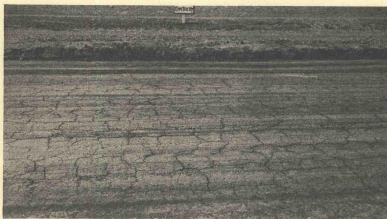
Figure 23. Rolling was not continued during drying period and stabilized base shows many shrinkage cracks which were closed by sprinkling and drag-brooming before construction of wearing surface.
