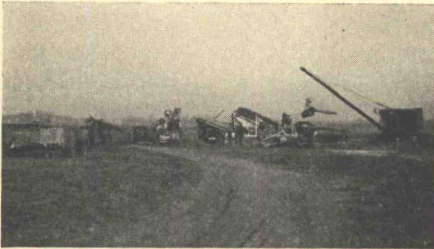
Figure 9. Plant for Producing Dry-Mixed Stabilized Road Material at Ames, Iowa
