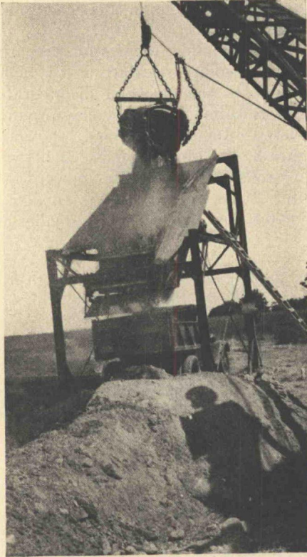
Figure 2. Vibrating Screen Breaking up Sand-Clay Binder-Soil
