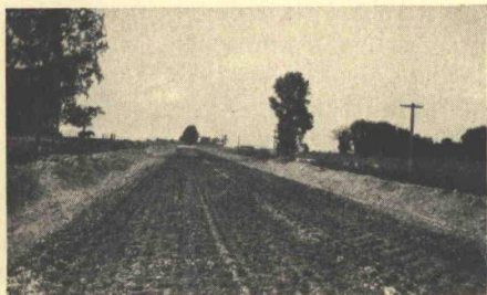
Figure 3. A view of stabilized road after being compacted with the sheepfoot roller. Eight and one-half inches of material were compacted to a 5 inch thickness. The course is then brought to the proper cross section and finish rolled.
