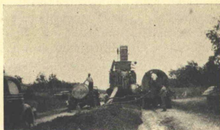
Figure 5. Traveling plant of the pug mill type used in mixing asphalt emulsion and gravel. The aggregate was picked up from a windrow and run through a pug mill at which time the emulsion was added. The mix was allowed to dry for about four days. It was then spread and compacted.
