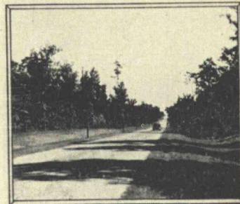
Bituminous surface treatment on U.S. Route 90, in Florida
