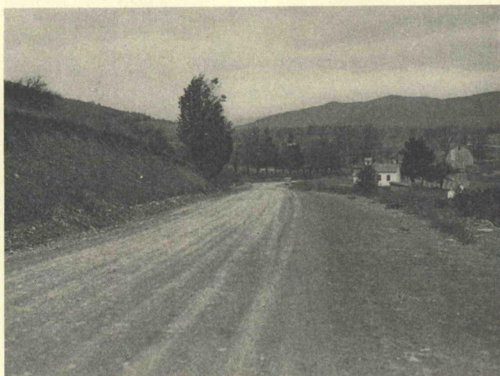
Figure 7. A Coarse Graded Mix with a Top Size of Approximately 2\frac{3}{4} In. In this Case Run of Bank Gravel Was Mixed with the Roadway Soil
