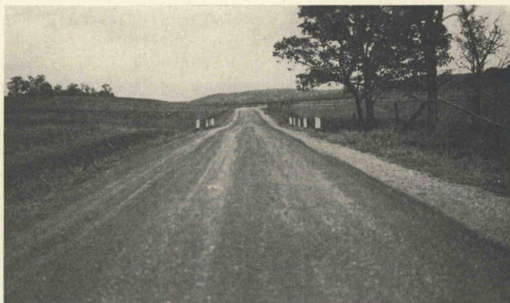
Figure 5. Coarser Mix, Top Size Approximately 1\frac{3}{4} In. Run of Crusher Slag, Including Fines, Was Incorporated with the Soil in the Roadway
