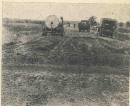
Figure 22. General view of turn-around and temporary wooden joint to be removed, after which the wet-mixed materials are pushed back into place. The length of the turn-around is about 30 ft. Missouri photo.
