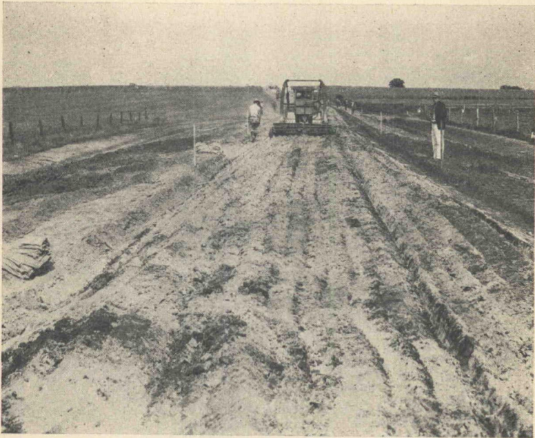
Figure 4. Mixing cement with the soil. Illinois photo
