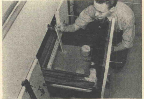
Figure 11. Technique of Making Heave Measurements
