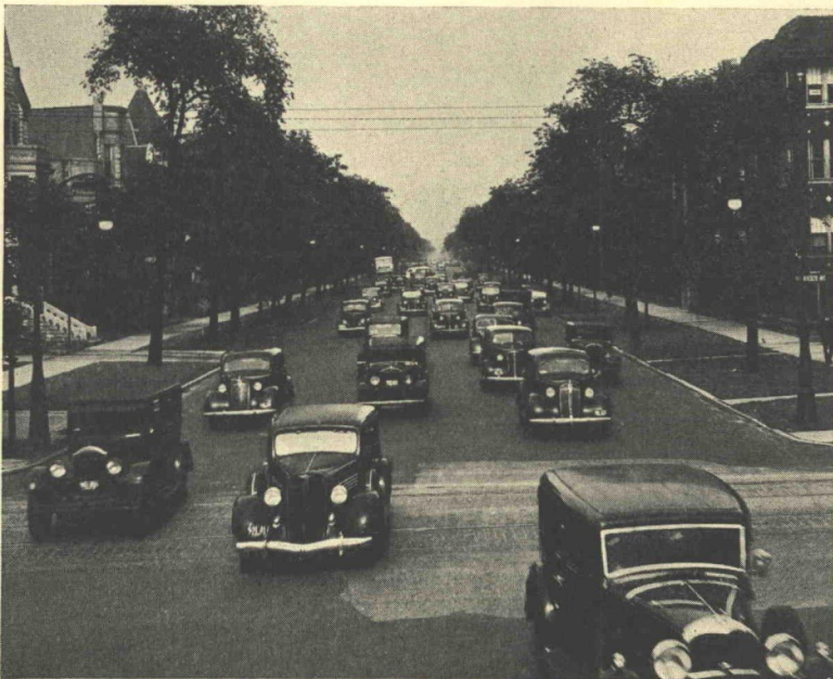
Figure 2. Washington Boulevard and Kedzie Avenue, Chicago. Looking East at 4:50 P.M.
