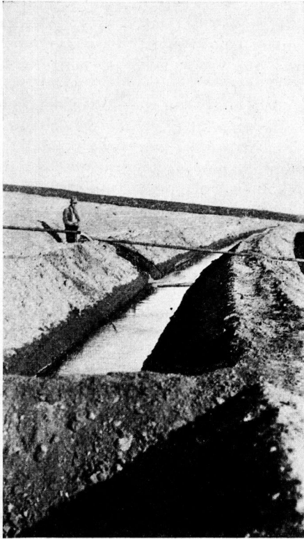
Figure 14. Irrigating a Hillside Borrow Pit Location in Norton County, Kansas. The moisture penetrated to a depth of 12 ft. in this silty loam soil.
