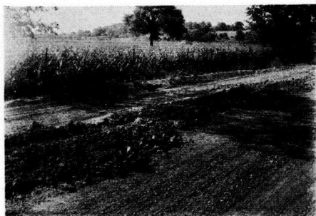
Figure 23. Binder-Soil Delivered on Roadway, Preliminary to Drying and Pulverizing
