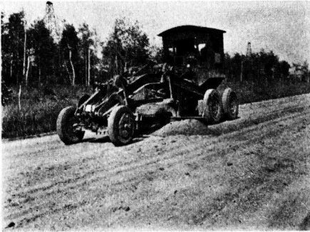
Figure 24. Mixing with Motor Grader
