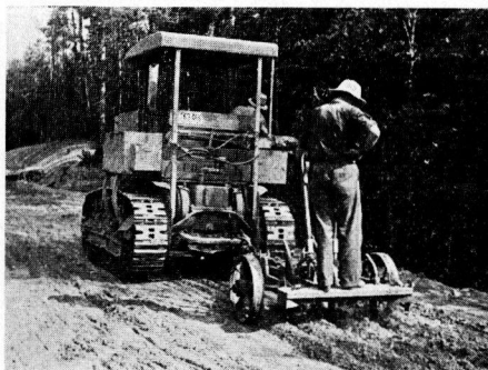
Figure 2. Scarifying Existing Roadway
