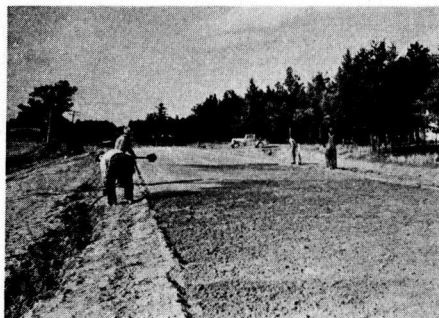
Figure 12. Protective Cover Permits Soil-Cement to Harden at Compacted Volume
