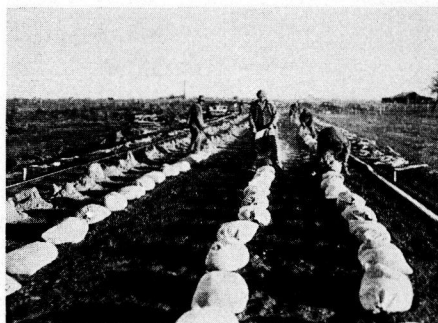
Figure 4. Applying Required Cement
