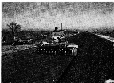
Figure 3. Pulverizing Roadway
