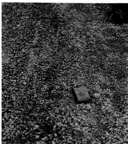
Figure 25. The Largest Shoulder Crack That Has Ever Been Found Where the Roadway Shoulders Are of Crushed Stone on Highly Expansive Clay Soil.
