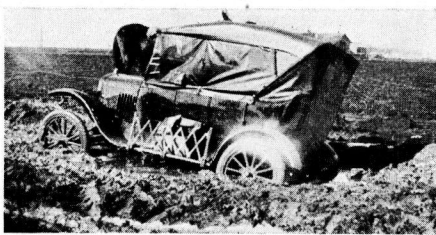
Figure 11. Exaggerated Subsequent Ill Effects of Placing Coarse-grained Material in a Trench Cut in Tight Highly Plastic Clay Soil.
