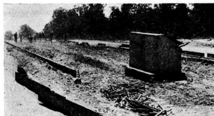
Figure 21. Effect of Setting Side Forms for Pavement so That the Wetted Excess Soil between the Side Forms Could Be Excavated to the Proper Subgrade Elevation without Appreciably Disturbing the Underlying Soil.
