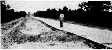
Figure 19. Irregularities in Pavement Surface Caused by the Subsidence of the Embankment When Water Was Ponded on It.
