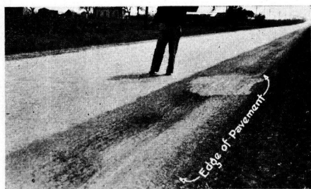
Figure 9. Showing Failures and Patching along the Edges of a Pavement Where the Crushed Conglomerate Base Material Was Placed in a Trench Cut in the Tight Clay Soil.
