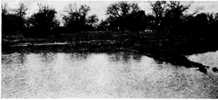
Figure 18. Ponded Water on a Soil Substructure Directly after Completion of the Grading Work.
