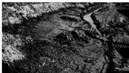
Figure 4. Drainage Conditions Encountered in a Sand Cut as the Excavation Approaches a Deep Substratum of Impervious Clay. This condition was corrected by means of open joint sewer and tile under drain. Michigan.
