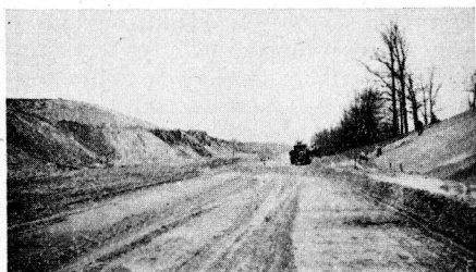
Figure 3. Materials for Backfilling Frost Heave Excavations May Be Found in the Same Cut. Note the unfinished bank of sand left for later use as subgrade material. Michigan.
