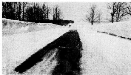
Figure 9. Snow Banks over Shoulders and Ditches Prevent Frost Penetration, and at the Same Time, Supply Capillary Moisture for the Freezing Subgrade. Michigan.
