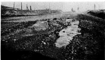
Figure 7. A Frost Boil Rupturing near the Edge of the Metal Permitting Escape of a Fluid Subgrade. Deep frost prevents a downward movement of water. Michigan.
