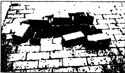
Figure 3. No Bond to Brick, Asphaltic
