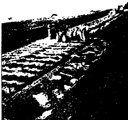
Figure 1. Cement sacks spotted and being dumped to form continuous transverse windrows, preparatory to leveling with spike tooth harrow.
