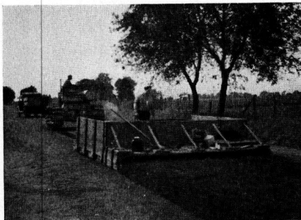
Figure 3. An inexpensive method of securing uniform distribution, of stabilized mixture. LaSalle County, Illinois.
