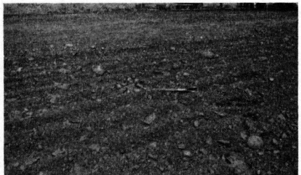
Figure 4. Oversized Stone Brought to Surface by Scarifying and Cultivating
