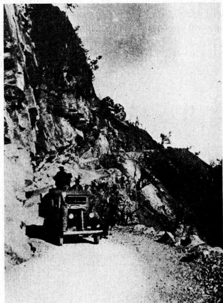
Figure 9. A Typical Rock-Cut Section of the Burma Road
