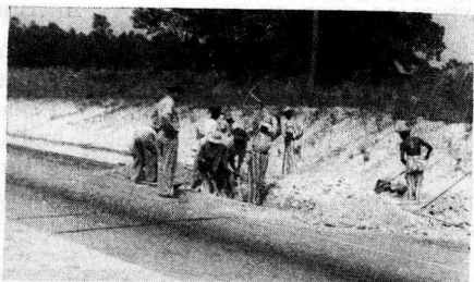
Figure 1. Removing old pavement and subgrade. The rigid pavement was broken with pneumatic tools, but subgrade was removed by hand.
