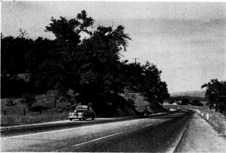
Figure 10. In dry climatic regions oiled shoulder surfaces like this may be desirable because good turf is all but impossible to grow. The same granular shoulder subbase provided here may also be essential on turf shoulders in humid regions.
