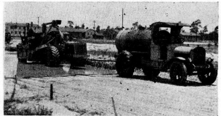
Figure 4. Tracking and Sprinkling Operations in Section 2.
