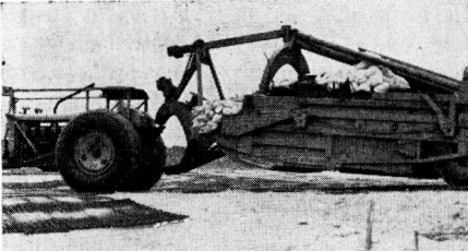
Figure 6. Large Tournapull Loaded to 60000-lb. Wheel Load.
