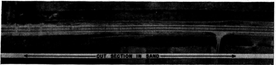
Figure 12. Good Pavement Performance on Sand Subgrade in Cut Section
