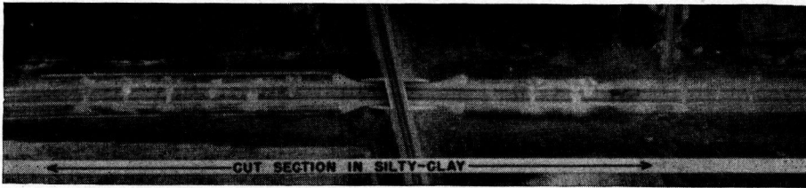
Figure 14. Poor Pavement Performance on Silty-Clay Subgrade in Cut Section—This section of pavement is adjacent to the location shown in Figure 12. The poor performance has been caused by pumping joints.
