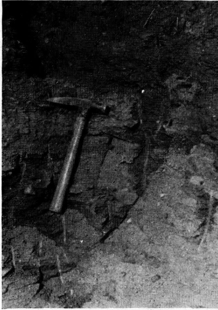
Figure 12. An Example of the Intense Fracturing Which is Characteristic of the Dense, Unweathered Illinoian Till. The high natural density of this material is an adverse factor in highway excavation.
