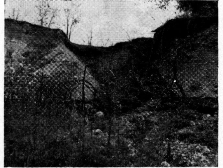
Figure 19. Gravel Gully. As long as the gully remains in granular soils it maintains its usual "V" shape. See location 7 or B-2, Figure 16.
