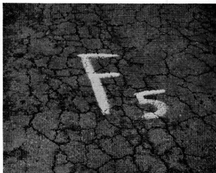
Figure 1. Base Failure
