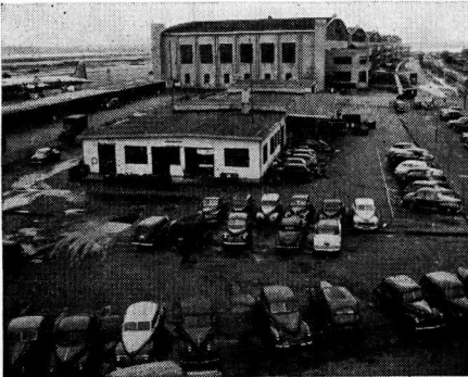
Figure 3. Where a Great Portion of Air Cargo is Handled Immediately Adjacent to Passenger Terminal
