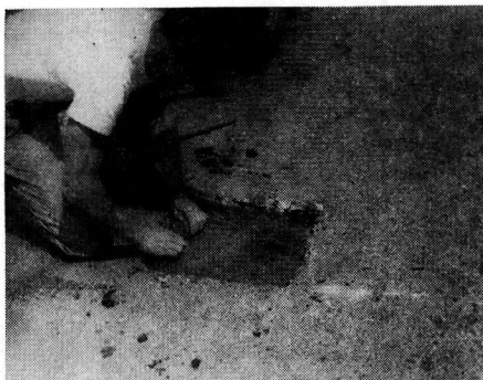
Figure 2. Removing Base Material Containing Prime and Leveling the Area
