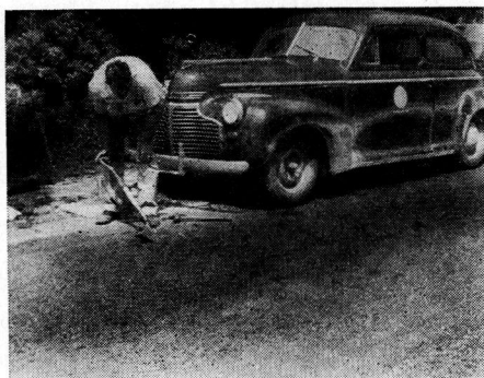
Figure 1. Removing Thin Bituminous Surface Treatment Mat
