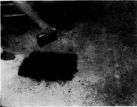
Figure 9. Sealing the Patch with Cut-Back Asphalt
