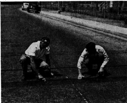
Figure 9. Installation Procedure: Applying the Protective Adhesive Tape Covering Over the Detecting Unit
