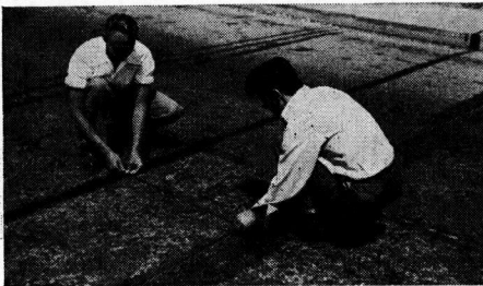
Figure 8. Installation Procedure: Locating the Detecting Unit for Speed Measurements
