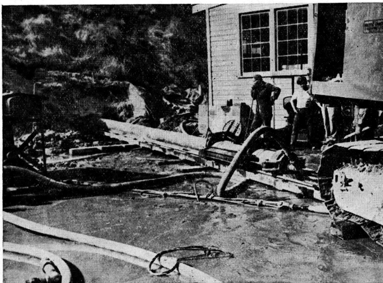
Figure 4. Jacking 12-In. Drain Pipe Into Embankment
