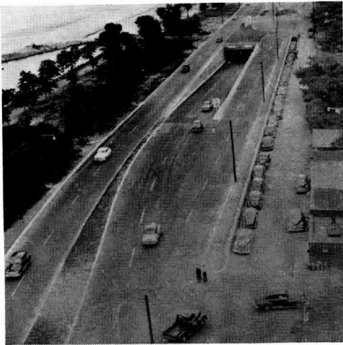
Figure 27. Massachusetts: Storrow Memorial Expressway in Boston.
