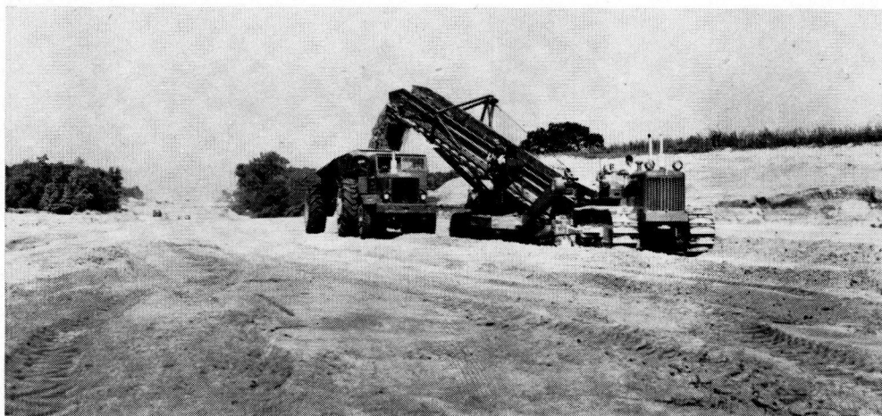
Figure 22. New Jersey: Construction on turnpike.
