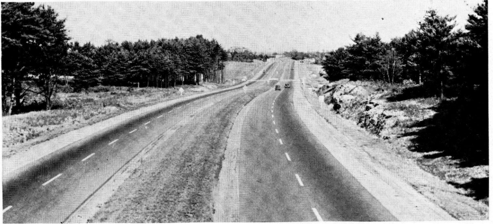
Figure 20. Maine: Section of Maine Turnpike.
