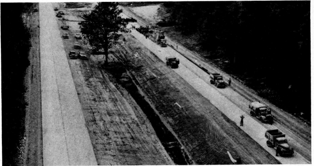
Figure 22B. New York: Section of thruway near Syracuse.
