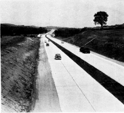
Figure 19. Pennsylvania: Eastern extension of turnpike.
