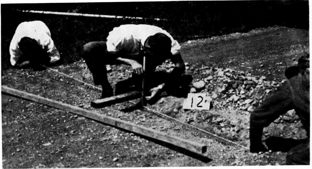
Figure 6. Trench measurements at Station 12.
