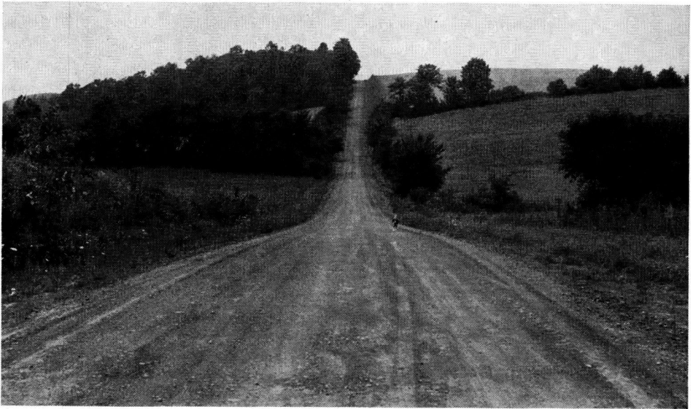
Figure 9. Sentinel Heights Road: 17 percent grade.
