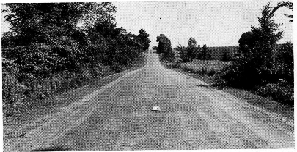
Figure 7. Station 18 on N. W. Town Line Road.
