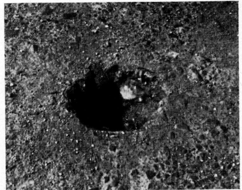
Figure 12. Test hole for density: Station 8.
