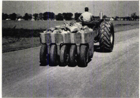
Figure 10. Pneumatic Rolling. This operation was begun during the final shaping of the blade-spread base.
