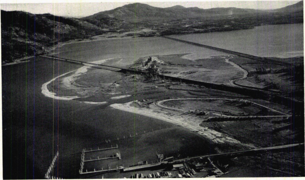
Figure 1. Highway bridge and railroad bridge and fill across arm of Lake Pend O'Reille.
