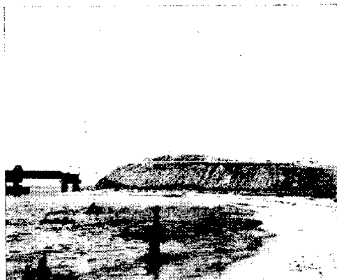
Figure 12. North plaza fill including 10-foot high surcharge and short length of 15-foot high surcharge.
