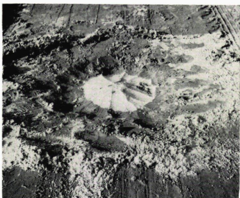
Figure 18. View of completed sand drain at fill surface.
