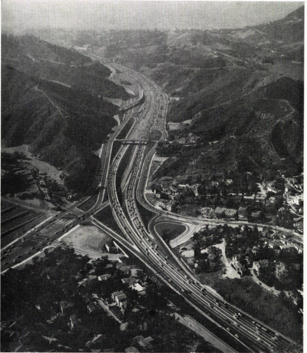
Figure 3. Hollywood Freeway looking northerly (outbound) through the Cahuenga Pass. Highland NB on-ramp (Location 22) in center. Mulholland Bridge (Location 13) in background. The 3-lane section (one-way) inbound (center, Location 14 and lower right, Location 47) carries a peak hour of 6,600 vehicles.
