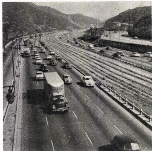
Figure 15. Location 13, Hollywood Freeway at Mulholland Bridge, at 4:12 PM, WB traffic during 4:11-4:16 period L_1 = 288 vph at 19 mph, L_2 = 1,332 vph at 33 mph, L_3 = 1,752 vph at 41 mph, L_4 = 2,196 vph at 42 mph.
