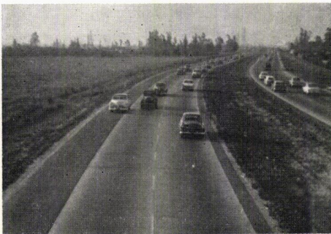
Figure 8. Location 7, Santa Ana Freeway looking southeast at Buhman Ave., 7:11 AM. Rate-of-flow WB during period 7:11-7:16: Lane 1, 1,512; Lane 2, 2,424. Note car passing on shoulder (less than 1 percent of vehicles counted did this).
