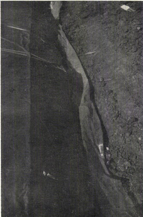
Figure 17. Edge of envelope, showing polyethylene and vinyl films ready for seal.
