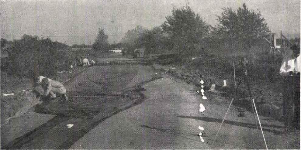
Figure 16. Placing 8-mil vinyl.
