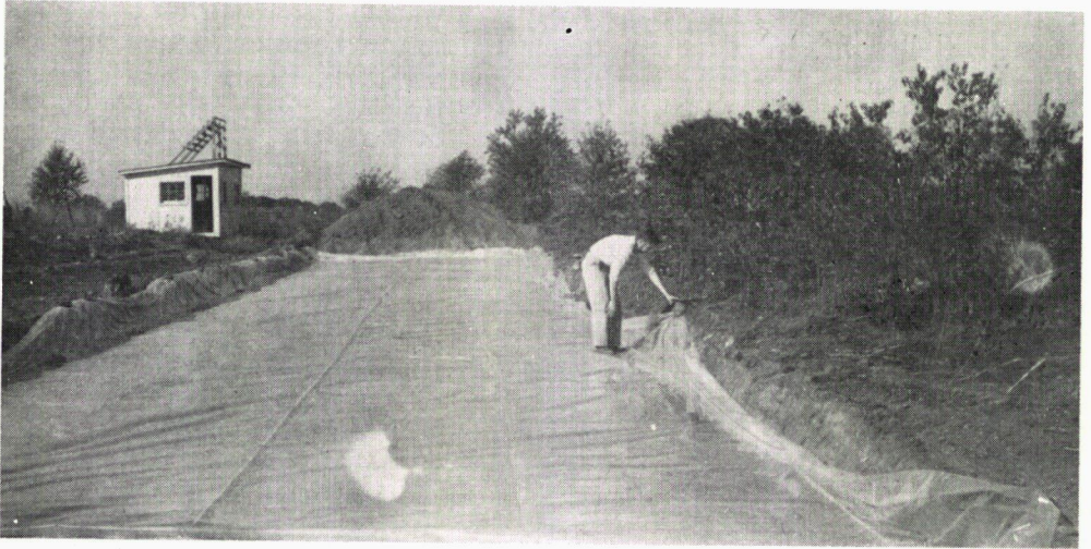
Figure 15. Polyethylene (4-mil) in place.
