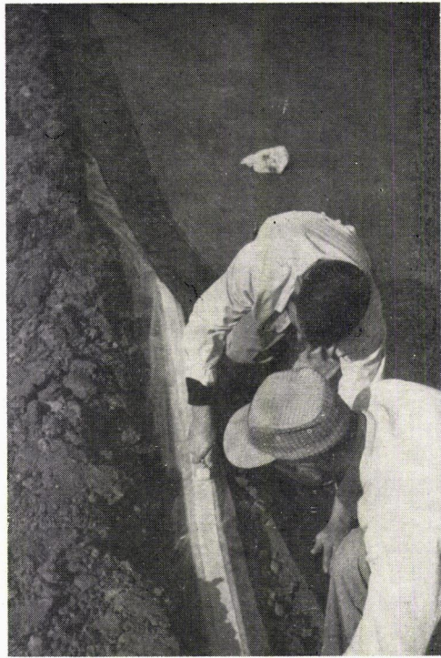
Figure 18. Sealing polyethylene and vinyl plastics with adhesives.
