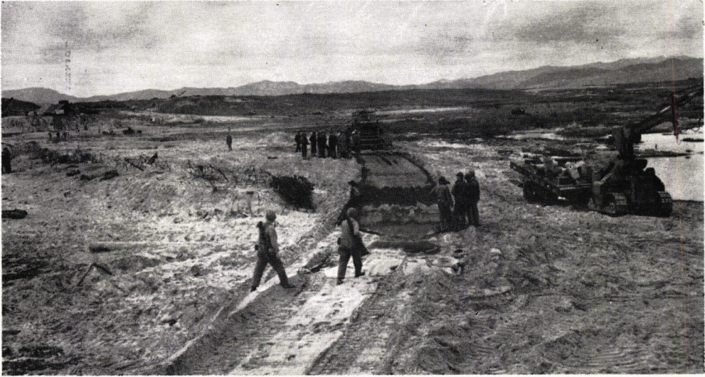
Figure 7. Use of traveling mixer in beach sand stabilization.
