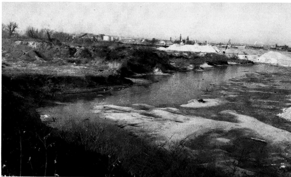
Figure 8. View of the gravel pit area before construction.
