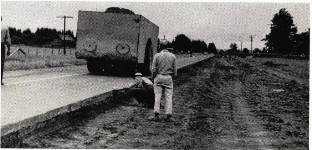
Figure 6. View of widening job with compactor on slab.
