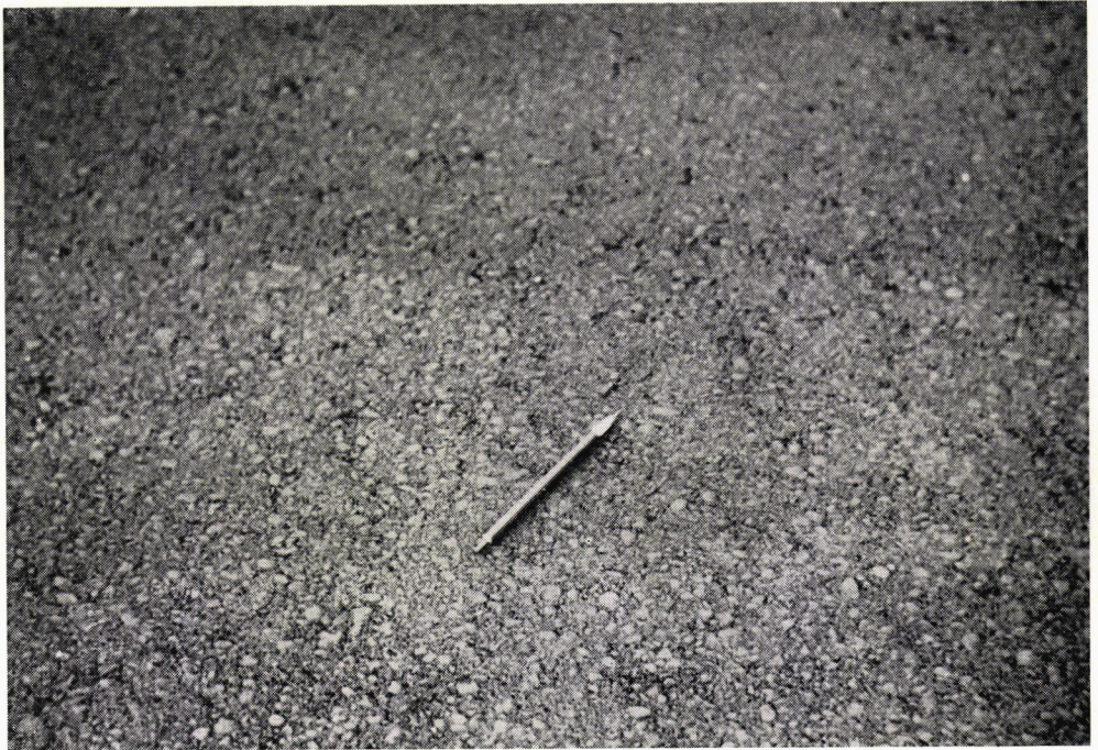
Figure 10. Wearing course of finished resurfaced pavement.
