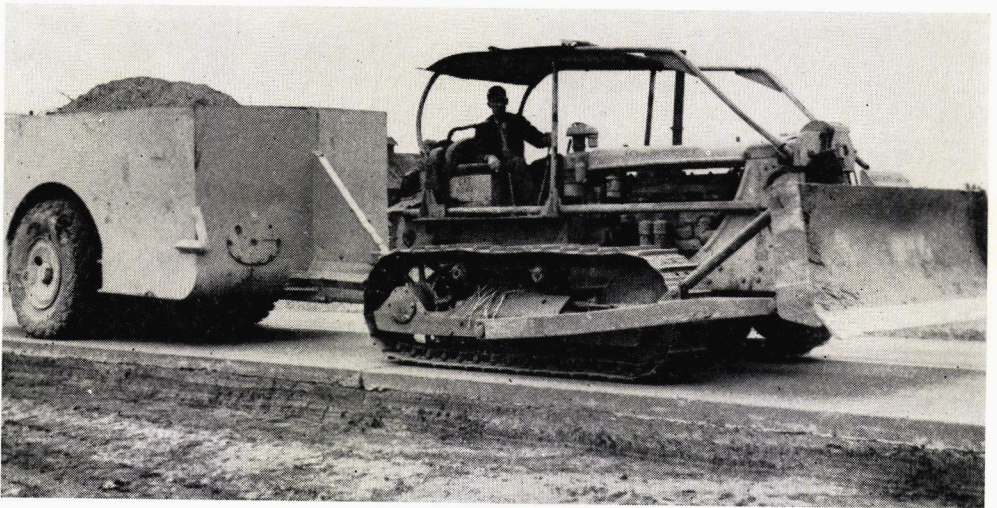
Figure 2. Compactor used to roll old slabs down to the subbase.
