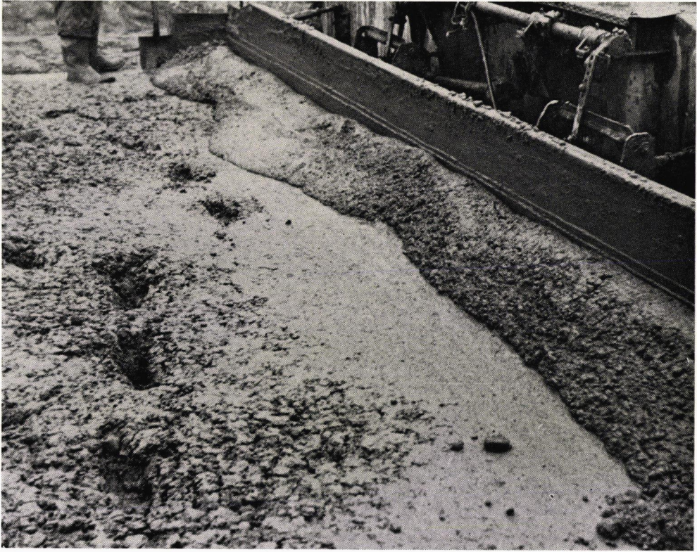
Figure 23. Typical appearance of air-entrained concrete.
