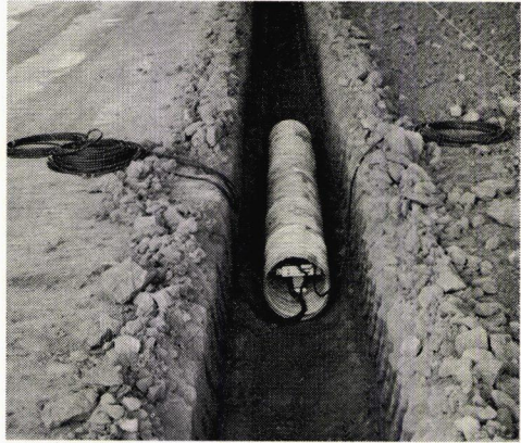
Figure 2. Test pipe in position before backfilling of trench.
