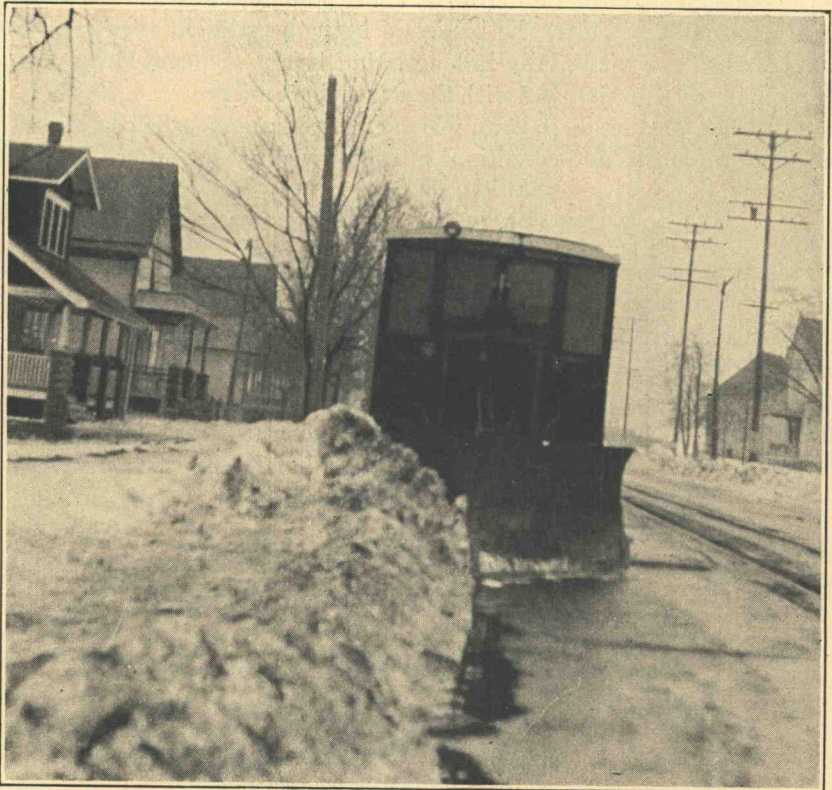
Figure 3—V-shaped plow on a truck
