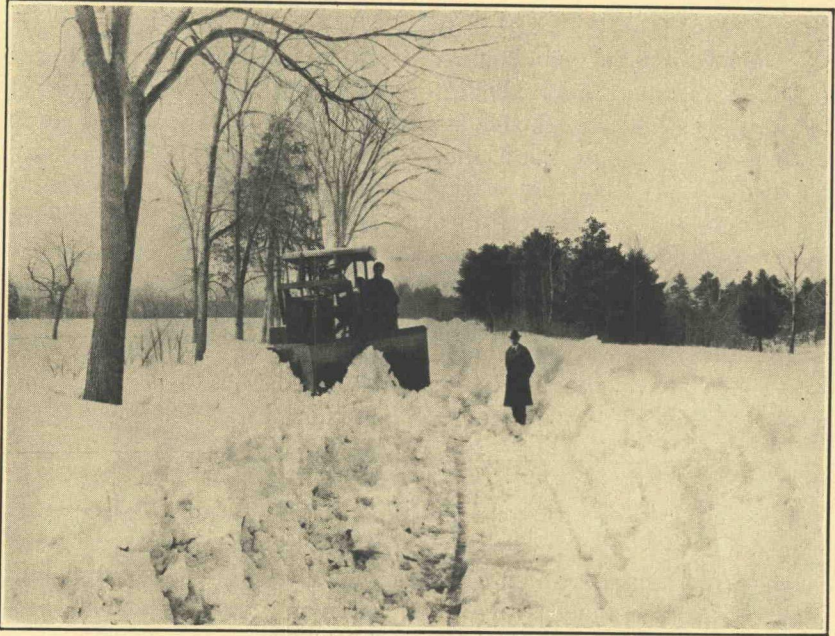
Figure 4—V-shaped plow on a tractor
