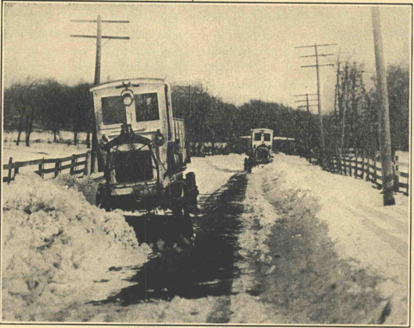
Figure 2—Pair of straight blade plows in action
