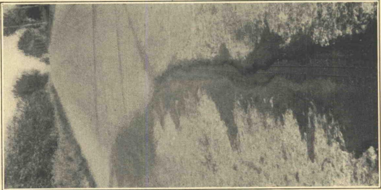
Figure 81—Open cracks in plain concrete slabs with side edge displacement
