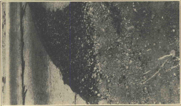
Figure 81—Open cracks in plain concrete slabs with side edge displacement
