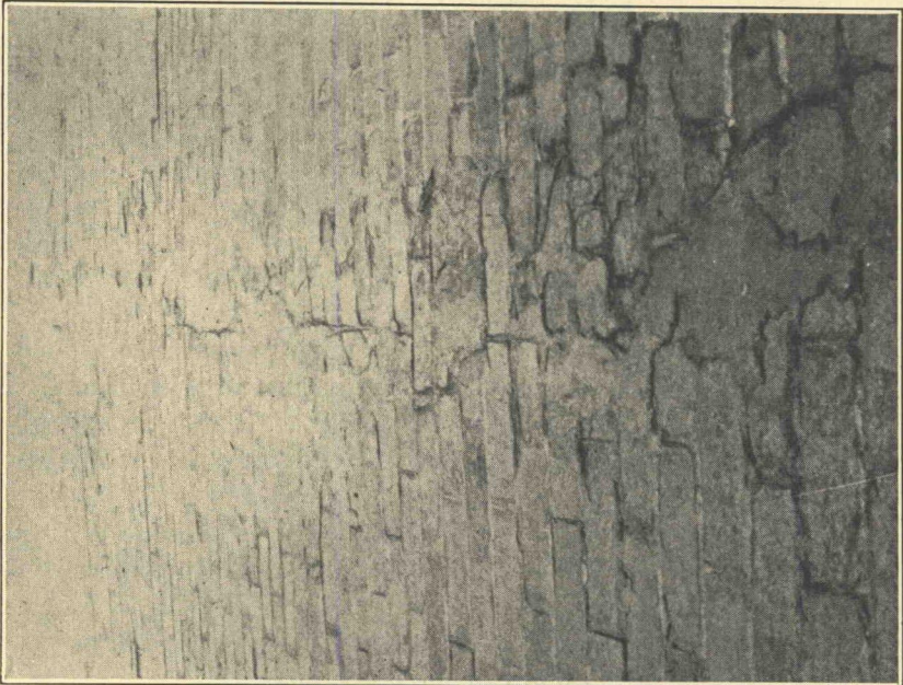
Figure 71—Brick tops on plain and reinforced bases Stations 327+59, Road No. 1066
