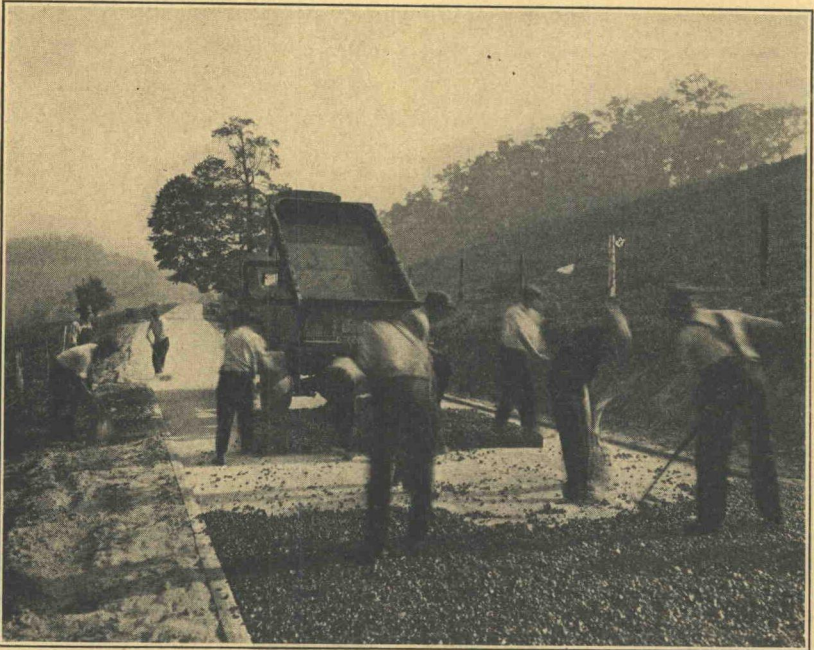
Figure 80. Premixed Bituminous Surface. Laid Cold. Dumping on Dump Board, Placing and Spreading. Pennsylvania
