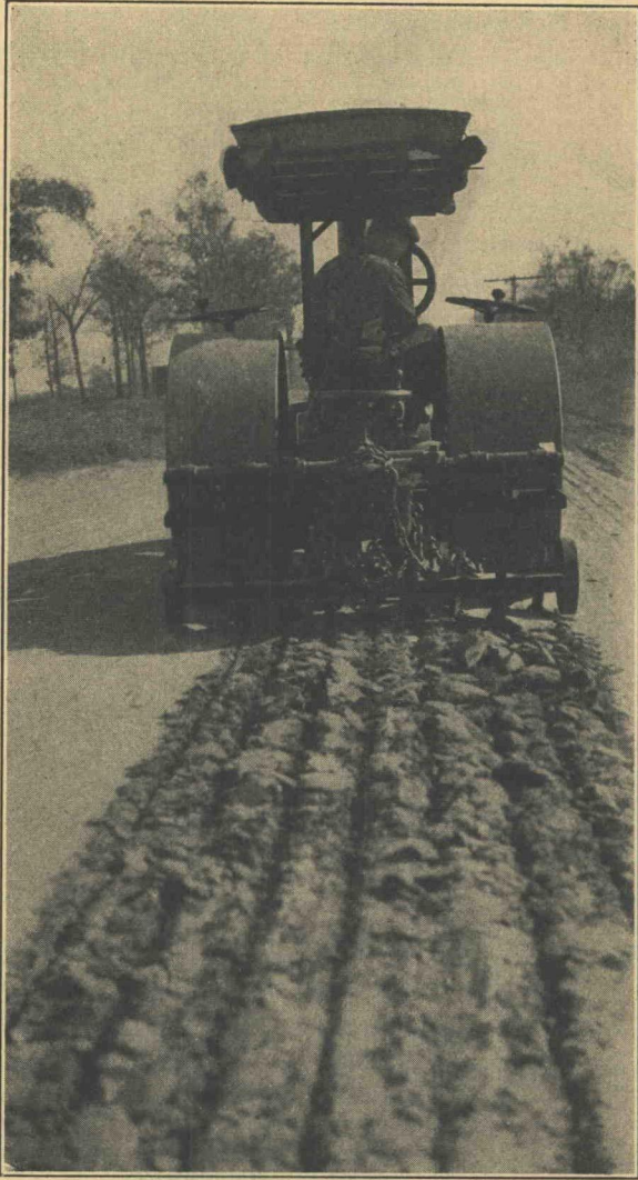
Figure 12. Scarifying a Well-Compacted Surface, Using a Light Roller with Scarifying Attachment
