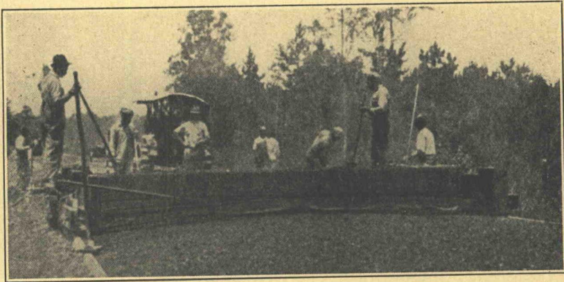
Figure 88. Mechanical Spreader and Finisher. Pre-Mixed Bituminous Surface Laid Hot. From Public Works, Vol. 59, No. 3
