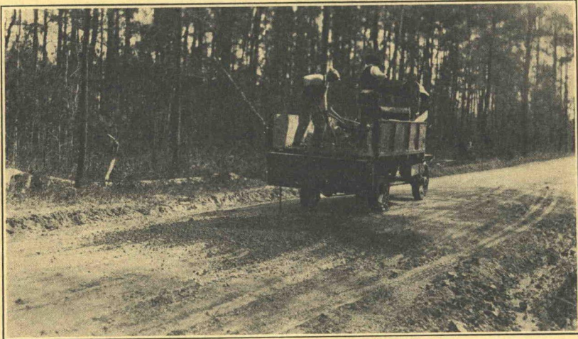
Figure 53. Patching a Sand-Clay Surface
