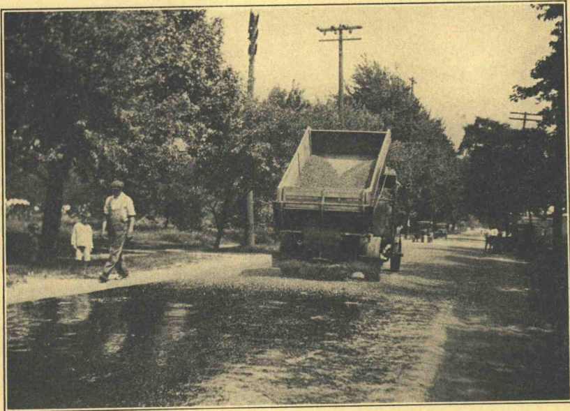
Figure 65. Distributing Slag over Bitumen. Bangert Distributor, Michigan
