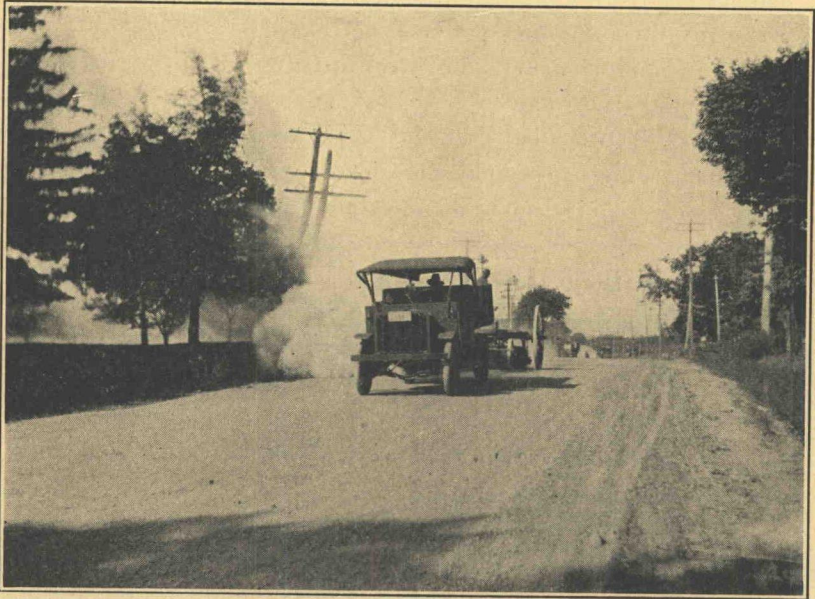
Figure 69. Dual Bituminous Surface Treatment. Sweeping Surface Before Bitumen Is Applied. Wisconsin
