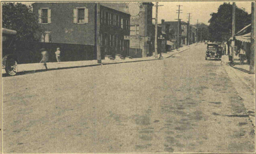
Figure 91. Water Bound Macadam Surface Maintained 7 Years with Tar and Sand Treatments
