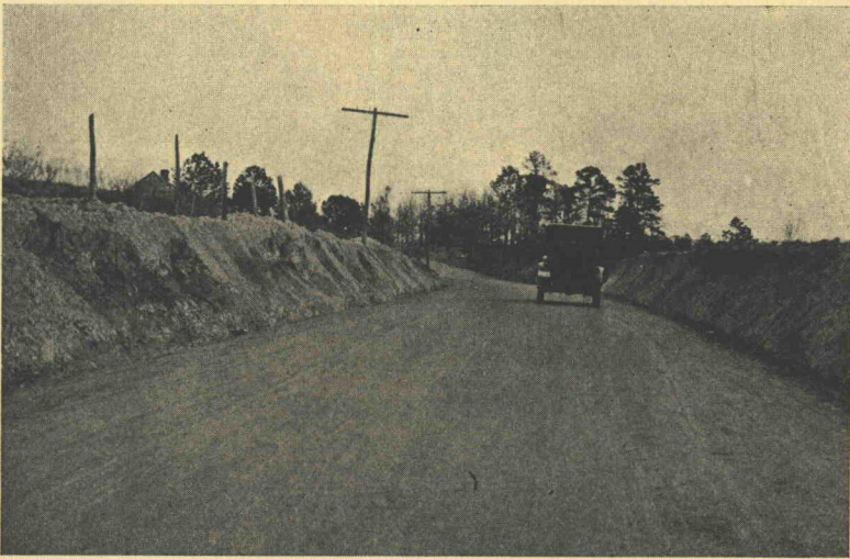
Figure 3. Highly Stable Mixture of Sand, Silt and Clay Possessing Both Internal Friction and Cohesion in Proper Amounts
