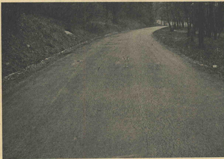
Figure 4. Detrimental Effects of Elasticity in the Subgrade
